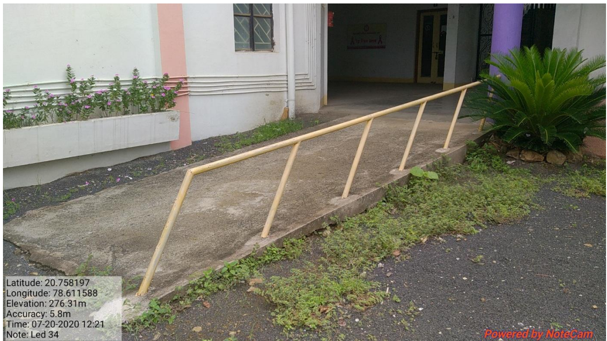
Figure 1 Ramp and Railing No. 2
