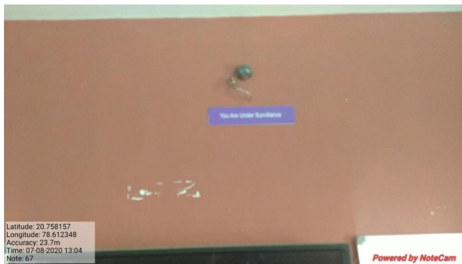
Figure 7 Room No. 2 - Camera 4
